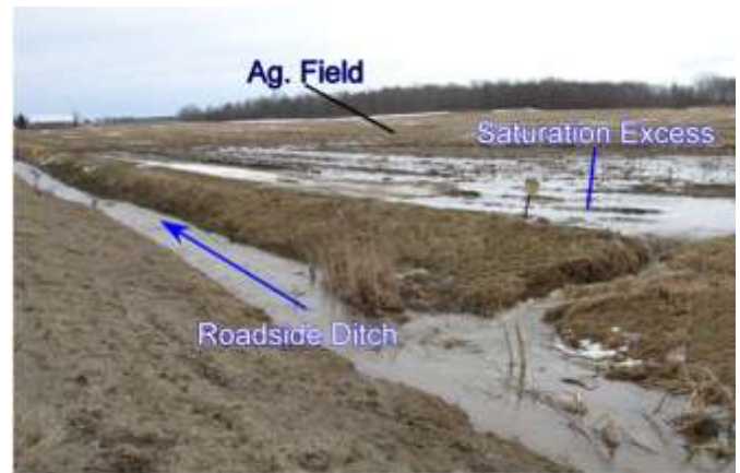
Typical VSA - agricultural field – roadditch interaction observed within the study region. Road ditch flow eventually discharges to a natural stream.
